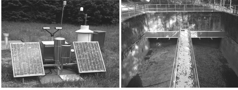
Figure 1: Left: rain gauge (pluviometer). Right: stormwater tank.
